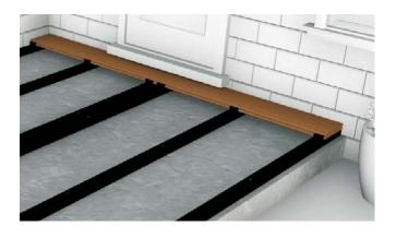
4 Fixing Clips are then slotted into the Boards groove on the side and screwed into your supporting Joists with Screws provided, an individual Fixing Clip is used per Joist. We suggest opting for our Stainless Steel Wood Screws due to their durability and reduced chance of corrosion. Between your Bamboo Decking Boards, Fixing Clips will give a 6-7mm break between Boards.
