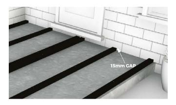
2 Before your first Decking Board is placed, a Starter Clip must be fixed on to the Composite Joists end. Starter Clips need to be placed at every Joist end where your Bamboo Boards will lay. A slight gap should be left between the Joist end and any walls.
