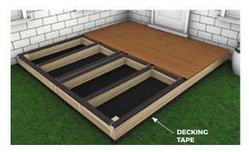
Slide the next Board onto the **Secured Fixing Clips from the first** installed Board, fit a Fixing Clip set to fasten the alternate side of your Board, a single Fixing Clip is to be used per supporting Joist. To fit the rest of the Boards, proceed with a similar method. Make sure the Decking Board ends are fully supported. It is advised to have no cantilever or overhana.
