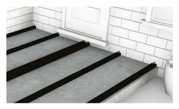
3 Our Bamboo Boards are fastened easily to supporting substructure Joists, our Fixing Clips and Stainless Steel Screws allow for simple installation. From the outer sides of your structure, lay your first Bamboo Board and, with a row of Starter Clips, fix on each Joist that it crosses.
