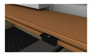
4 In the groove across the edge of the Bamboo Board, position Fixing Clips and screw into supporting Joists using Screws provided, for every supporting Joist use one Fixing Clip. Our Stainless Steel Wood Screws are recommended as they offer increased durability with less corrosion. A 6-7mm gap between Decking Boards is created by Fixing Clips.
