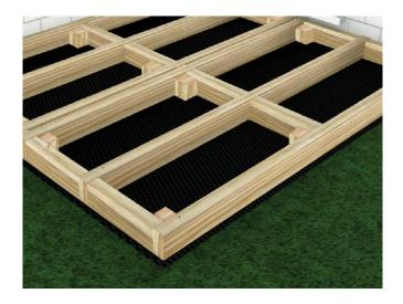
We recommend leaving a space of **450-500mm between rows of Joists**. Deck Tape can be applied and to protect Timber Joists from moisture at cut the ends. For raised Decking areas, ensure Posts are placed at 1m intervals across the installation for adequate support.
