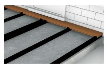
Each Board should be held into place with a Fixing Clip where two Board ends meet. Allow 2mm of spacing between butt joints.
