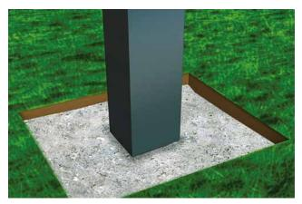
Make sure every Fence Post is 100% level before using postcrete. Fence Posts must have at least 25% of their height concreted into place.
