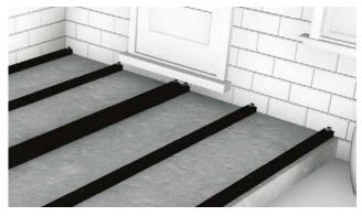
A Starter Clip needs to be fixed to the end of the composite Toists before law. composite Joists before laying the first board. Place these at the end of each Joist where you will start to lay your Boards, leaving a gap of 15mm between the wall and the end of the Joist to allow for expansion.
