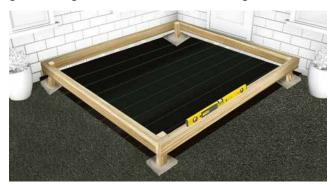
If your deck will be sitting on grass or soil, you will need to place blocks or slabs underneath each leg, to spread the load and provide a level, stable base. Additional blocks can be used if required. Position and adjust the blocks/slabs, ensuring the frame is at a slight angle, that will allow the water to drain down the length. We recommend a slope of at least 5mm for every metre. Alternatively, if using slabs, you could dig a hole and set the legs in concrete.
