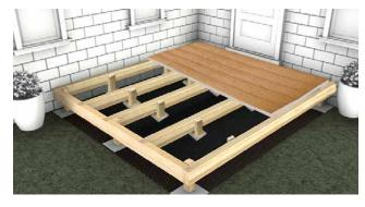
**7** Start by laying out your Decking Boards onto I the desired area before fixing them in place. Ensure there is a 3mm gap between any boards at butt ends or side by side and between all walls and fences.
