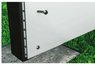
When adding the first Fence Panel Board, ensure  $oldsymbol{ extstyle 0}$  it is 100% level before fixing to posts. Screw the top and bottom of each Fence Panel to the Fence Posts behind.
