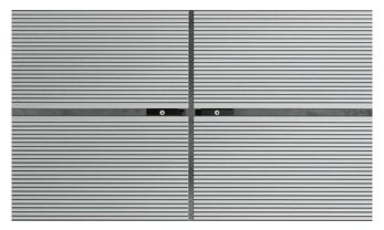
**5** Fit your next Board by sliding it onto the T-Clips used to secure the first Board and fitting another set of T-Clips to secure the opposite side of the Board, using one T-Clip for each supporting Joist. Follow a similar process to fix subsequent Boards. The ends of Boards must be fully supported. No overhang or cantilever is advised.
