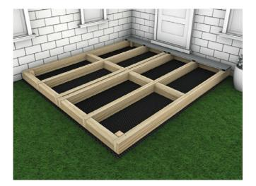
**3** Our Composite Boards are easily fastened to the Joists of a supporting substructure with the help of our Stainless Steel Screw and plastic T-Clip System. Start at the outside of the area to be decked. Place your first Board and fix it to each Joist it crosses using a row of Starter Clips.
