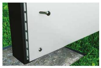
3 When adding the first Fence Panel Board, ensure it is 100% level before fixing to posts. Screw the top and bottom of each Fence Panel to the Fence Posts behind.
