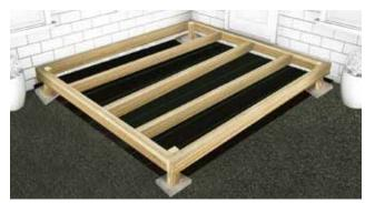
**5** Measure across the inside of the frame at your joist marks, then cut lengths of (47mm x 100mm or 47mm x 150mm) timber to suit. To fix the joists, tap them in with a hammer, until flush with the top, ensuring they do not push the frame out of shape. Then screw them in place from the outside of the frame.
