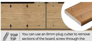
You can use an 8mm plug cutter to remove sections of the board, screw through the board and then replace with the section removed on top of the screw.
