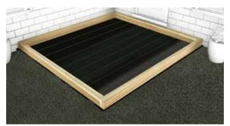
Prepare a level, weed-free area for the deck. To create a framework, cut the joists (using either a 47mm x 100mm or 47mm x 150mm) to the required length, then join using exterior wood screws. Check the frame is square, by measuring diagonally from corner to corner. If installing on grass or soil, use a weed mat to ensure weeds do not grow through from the base of the decking frame.
