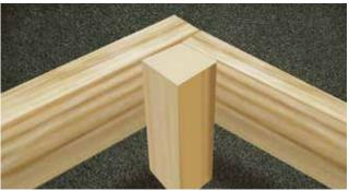
2 To raise the frame, cut four blocks of 100 x 100 treated timber, to the desired height. Screw these to the inside of the frame, at each corner, ensuring they are flush with the top. These legs will be taking all the weight for now, so ensure they are properly supported using blocks and secured to the frame.
