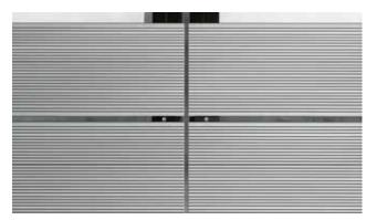
At butt joints - where the ends of two Decking Boards meet, this may mean doubling up on supporting Joists as you will need to ensure that each board is held in place with its own T-Clip where they meet.
