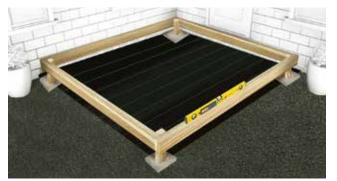
J If your deck will be sitting on grass or soil, you will need to place blocks or slabs underneath each leg, to spread the load and provide a level, stable base. Additional blocks can be used if required. Position and adjust the blocks/slabs, ensuring the frame is at a slight angle, that will allow the water to drain down the length. We recommend a slope of at least 5mm for every metre. Alternatively, if using slabs, you could dig a hole and set the legs in concrete.
