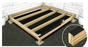
5 Measure across the inside of the frame at your joist marks, then cut lengths of (47mm x 100mm) or 47mm x 150mm) timber to suit. To fix the joists, tap them in with a hammer until flush with the top, ensuring they do not push the frame out of shape. Then screw them in place from the outside of the frame. Apply Deck Tape to the top surface and cut ends of joists to protect them from moisture.
