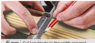
Cut two blocks to the width required **TOP** and use this as spacers for the joists.
