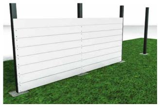
As you start to add more boards ensure each As you start to add more fixing. Each fence panel is 100% level before fixing. Each Fence Panel slots on top of the board previously fitted. (Example shows 3.6m fence panels with Fence Post in between).
