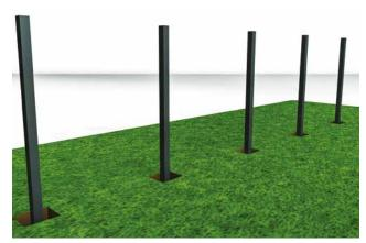
Prepare your area by removing any stones, debris or hazardous material. Dig the Fence Post Holes to 25% of the post height. The Fence Posts must be a maximum of 1.6m apart to ensure they can support the Fence Panels.
