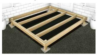
Measure across the inside of the frame at your joist marks, then cut lengths of (47mm x 100mm or 47mm x 150mm) timber to suit. To fix the joists, tap them in with a hammer, until flush with the top, ensuring they do not push the frame out of shape. Then screw them in place from the outside of the frame.
