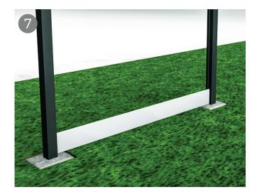
When using the cut method the fence panels need to be cut into 2 metre lengths. The posts must be no further apart than 2 metres.
