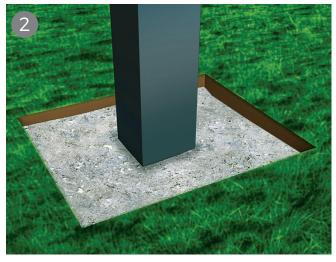
Make sure every fence post is 100% level before using postcrete. Fence posts must have at least 25% of their height concreted into place.
