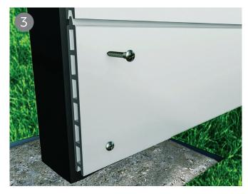
When adding the first fence panel board, ensure it is 100% level before fixing to posts. Screw the top and bottom of each fence panel to the fence posts behind.
