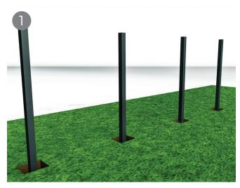
Prepare your area by removing any stones, debris or hazardous material. Dig the fence post holes to 25% of the post height. The fence posts must be a maximum of 2m apart to ensure they can support the fence panels.
