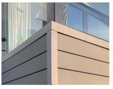
Cladco Composite Fascia Boards can be installed using both Sumo Grip Adhesive and 50mm Speeddekz Screws. When installing alternate between Sumo Grip and Screws every 150mm until the Board is firmly in place. The supporting structure underneath the decking must have adequate supports for the fascia board to be secured into. Sumogrip alone will not support the weight of the board and must be used in conjunction with screws.
