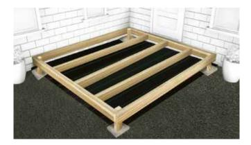
A Mark across one side of the frame every 300mm, this will set your joists at the recommended required 300mm centres, then repeat the process on the opposite side of the frame. You may wish to set your joists at smaller than 300mm centres, to ensure even spacing of the joists across the frame. Remember you will need to have a double joist in areas, where the ends of two boards meet.
