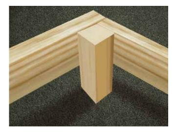
2 To raise the frame, cut four blocks of 100 x 100 treated timber, to the desired height. Screw these to the inside of the frame, at each corner, ensuring they are flush with the top. These legs will be taking all the weight for now, so ensure they are properly supported using blocks and secured to the frame.
