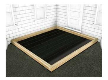
Prepare a level, weed-free area for the deck. To create a framework, cut the joists (using either a 47mm x 100mm or 47mm x 150mm) to the required length, then join using exterior wood screws. Check the frame is square, by measuring diagonally from corner to corner. If installing on grass or soil, use a weed mat to ensure weeds do not grow through from the base of the decking frame.
