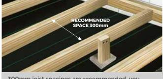
300mm joist spacings are recommended, you should never exceed 400mm spacings.
