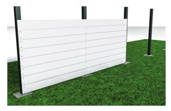
As you start to add more Panels ensure each Panel is 100% level before fixing. Each Fence Panel slots on top of the Panel previously fitted. (Example shows 3.6m Fence Panels with a Fence Post in between).
