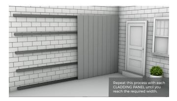
It is possible to fit your Boards side by side by simply butting the two ends up together. You may need to install more Battens if you wish to do this, as each Board will need to be supported on a Batten where it meets the next Board. Continue to fit the Cladding Boards in this manner until you have completely covered the area you want.
