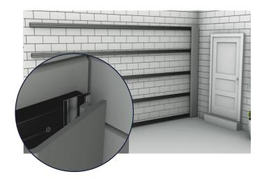
Place the first Wall Cladding Board on to the Starter Strips. Mark and then pre-drill pilot holes through the fixing groove of the Board into the Composite Batten below. Secure the Boards using a screw at least 30mm in length, ensuring that the Board is fastened securely on each Batten that it touches. Secure these fixings by hand, as it is important not to overtighten the screws and risk splitting the Board.
