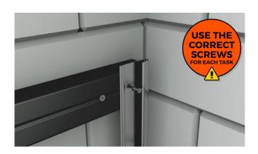
4 Attach a Starter Strip to the right side of each Batten, as this will give the first Cladding Board something to sit on. You may wish to pre-drill a pilot hole into the Composite Batten and attach the Starter Strip using a screw that is at least 15mm long. Ensure that each Strip is level with the next and that the first Board sits level on the Strips before continuing to the next step.
