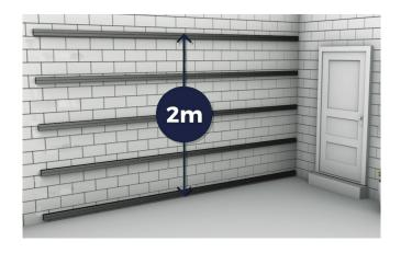
**Z** Battens should be attached to the **>** surface at a maximum distance of 500mm apart. The Battens will need to run the entire length of the area being clad, adding in additional Battens at any point where you will need to join two Cladding Boards end to end. Remember to install your Battens at a 90 degree angle to the way that you want your Wall Cladding Boards to run. It is important that the surface below the Battens is flat and stable.
