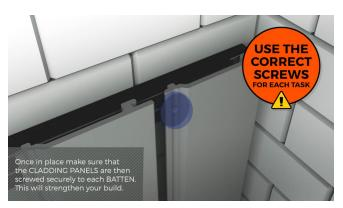
Ensure that the section between 6 the Battens remains empty allowing air to flow beneath the Boards. Slot the second Board onto the first and repeat the fixing process ensuring that the second Board is fitted securely in place on each Batten.
