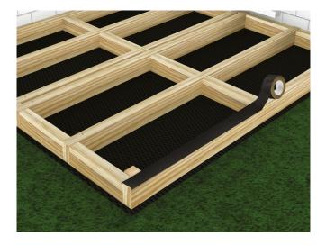
We recommend leaving a space of 45-50cm between rows of Joists. Deck Tape can be applied and to protect Timber Joists from moisture, cut the ends.
