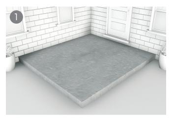
Step 1, Structural joists can be laid on top of a solid concrete base or a level area with weed mat covering. Make sure that the area to be installed on is flat and stable. If using a concrete base it should be at least **10cm thick** and have a slight slope – we suggest **a gradient of 1 in 80** – that runs away from the property to allow for the run-off of water that collects under the deck.
