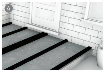
Step 4. If looking to use a raised decking frame area off the floor (something you can't easily step up onto) then use a 100mm x 100mm post every 1m and concrete the post into the ground or fix the post securely to the ground.
