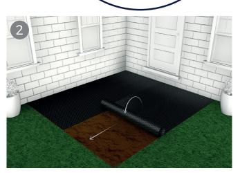
Step 2, Remove the turf until the ground is completely even. Cover the area of your site with a layer of weed control fabric to prevent any weed regrowth coming up under your decking. You may need to cut the weed mat to fit. You may want to pin your weed mat down at this stage.
