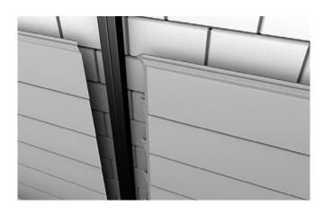
When butting two Boards together, you should use a mitered edge for a neat finish. The most common miter angle is 45 degrees. As the cuts are angled, you'll have one side of the wood longer than the other. You'll need to keep track of which side will be which and make your measurements correctly.
