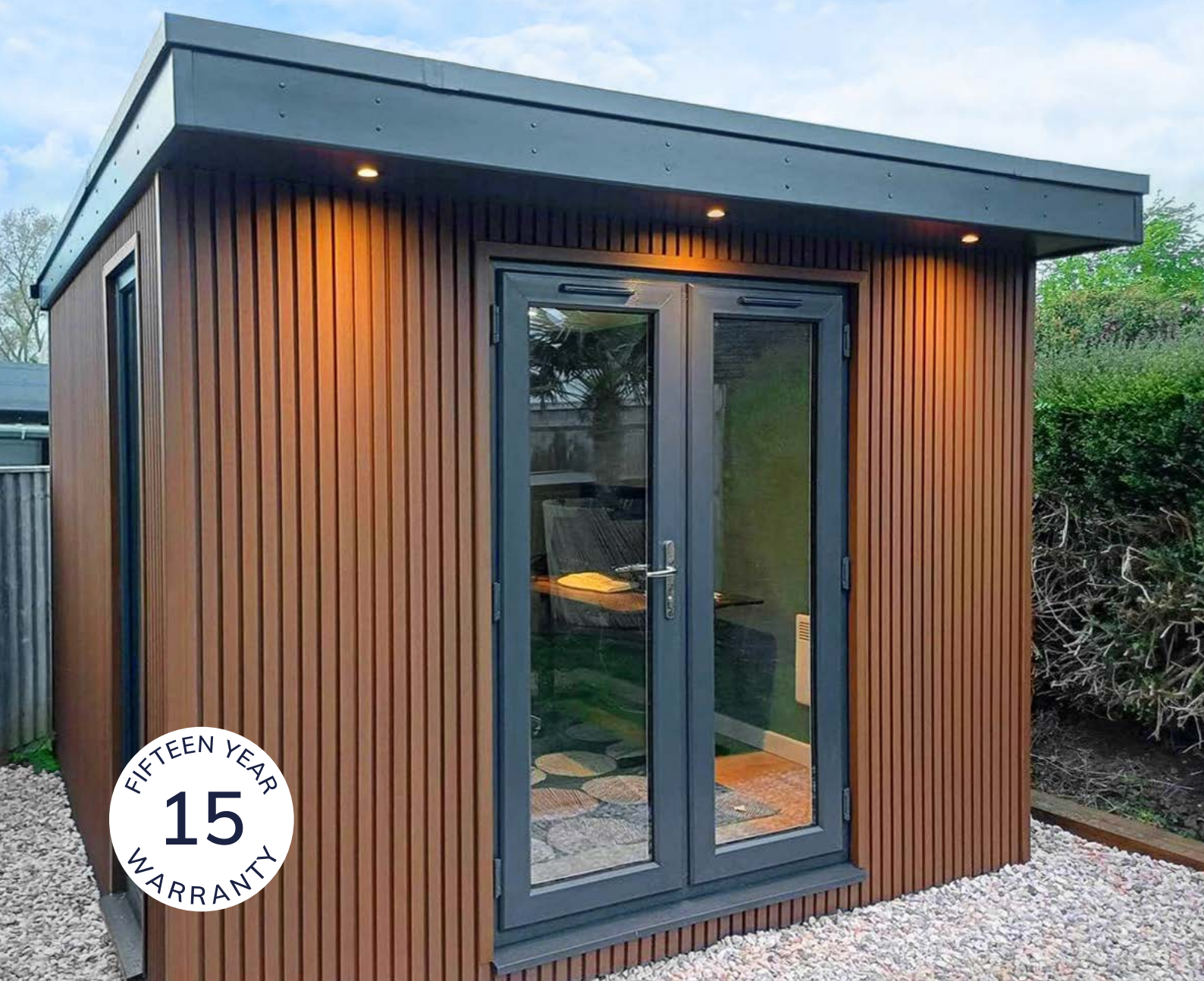
Pictured - Teak External Slatted Cladding
