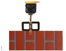
You will need to pre-drill the battens and the surface below using a 6mm drill bit, the battens are 30mm high and you will need to secure them at least 50mm into the surface below. You will need to choose fixings suitable for the surface you are fixing into. Screws should be 5-6mm diameter and at least 80mm long \*
